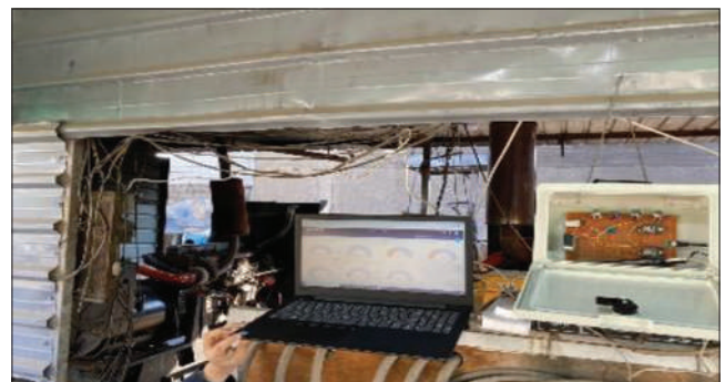
Figure 17: APM at the generator
