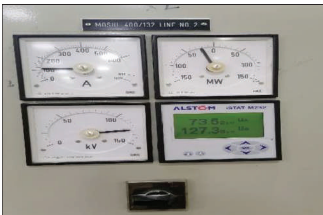
Figure 7: Gauge of voltage at the station
