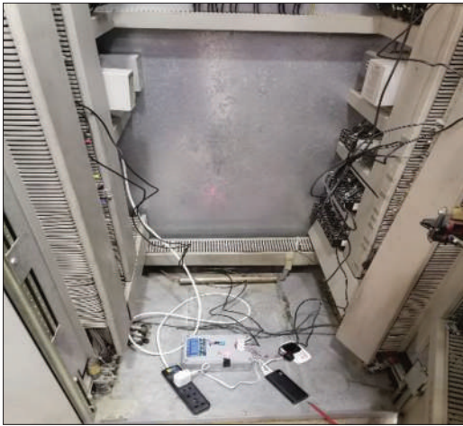
Figure 6: Connecting the device in the substation
